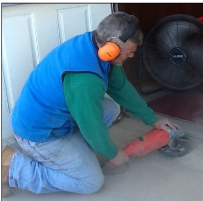
Contractor Phil Robles grinds down the lip at the front side door to help lessen the chance of someone tripping.
